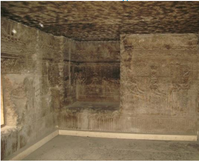
Half-staircase room, with niche
